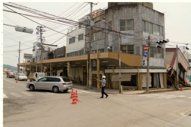
信号が止まった交差点 / Stopped traffic lights at an intersection
